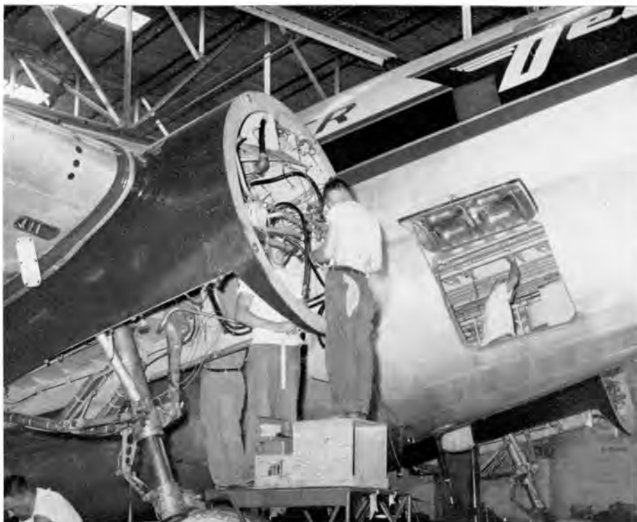
Delta mechanics at Miami are shown at work on the new C-46's. After preliminary modifications were completed at Civil Air Transport headquarters in Formosa, the freighters were flown to Miami for additional improvements.
